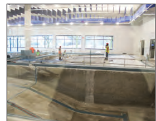
Swimming pools - in progress
