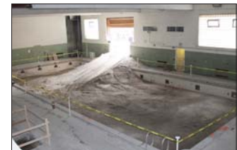
Filling in the swimming pool
