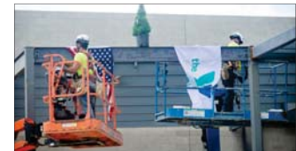
Planting the last beam
